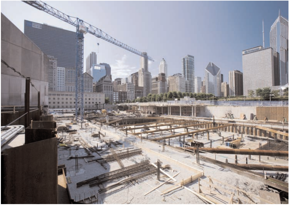
View of the Modern Wing under construction at the corner of Monroe Street and Columbus Drive.
